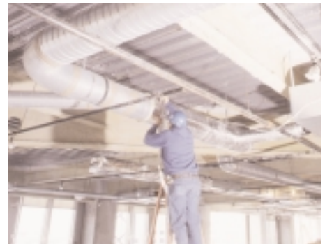
Closed cell foams are mostly used as external thermal wrap.
