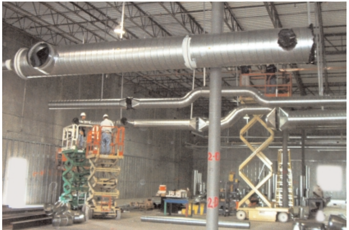
Using manifolded spiral ductwork reduced installation time and costs.
