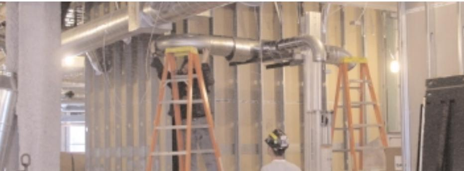
**McGill AirFlow's UNI-GASKET self-sealing ductwork was a "huge benefit" to HVAC contractor Central Ohio Sheet Metal: It is automatically sealed during the initial installation. There's no need to go back to seal it or fix leaks.**
