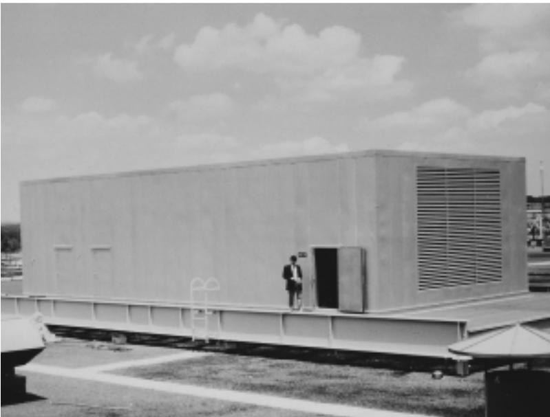
UNI-HOUSING enclosure utilized on a rooftop air conditioning application
