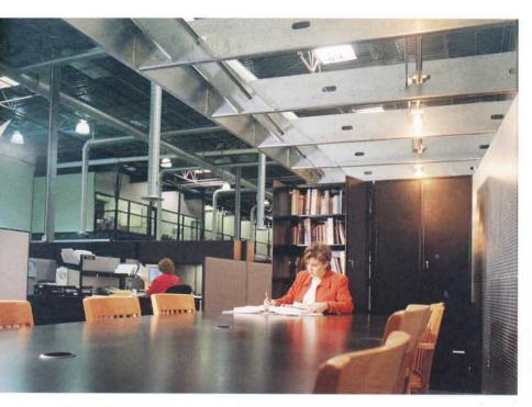
McGill AirFlow worked with Corn States Metal Fabricators to create a duct system with an industrial look that effectively heats and cools a large, open area.
